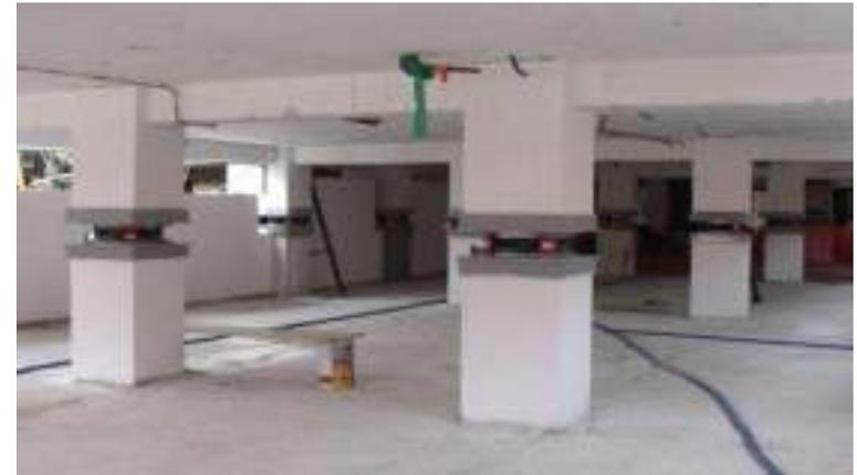
EXEMPLE D'UN RENFORCEMENT PAR ISOLATION
