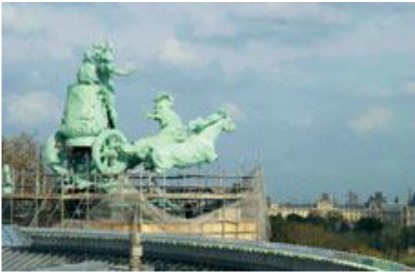
Vinci - Construction sites
